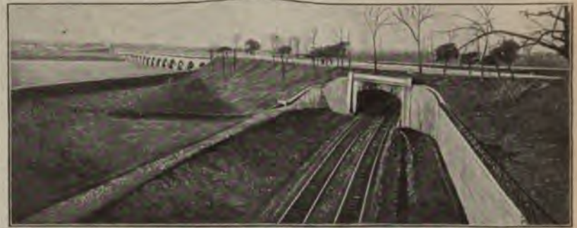
On the plain, southwest France, showing the river Garonne, a railroad, and a canal which is carried across both by an aqueduct bridge.
